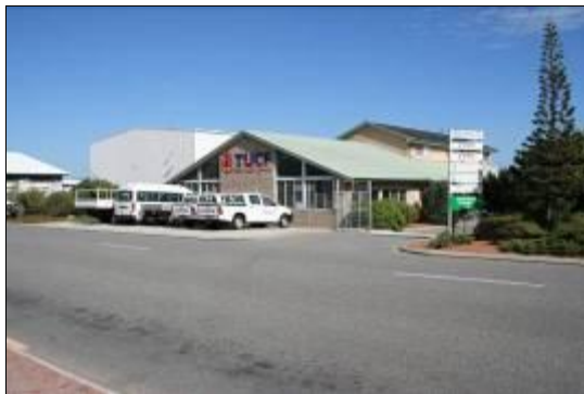
TUCF training facility in Rous Head, Fremantle.
